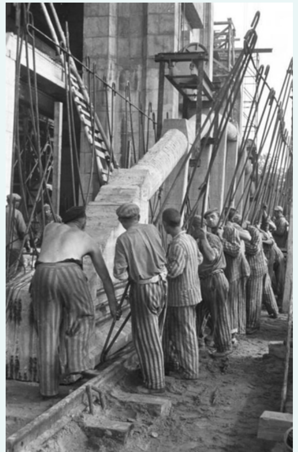
Prisoner work force in the construction.
